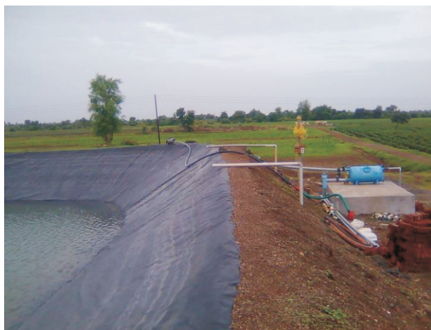
Pic.3 : Water supply to the Farm Pond From wells
